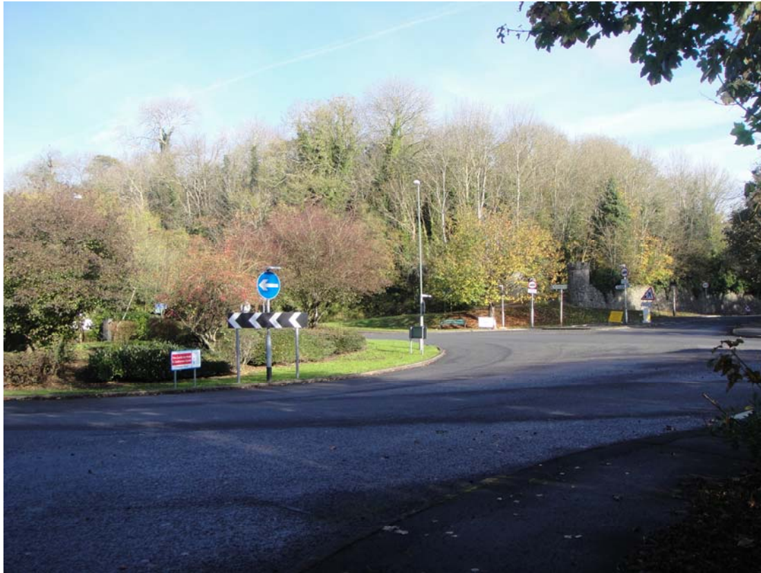
Figure 9: A283/A2037 roundabout looking towards Bramber Castle and St Nicholas Church
